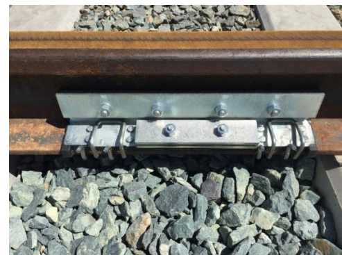
Tuned Dampers on ballasted track
