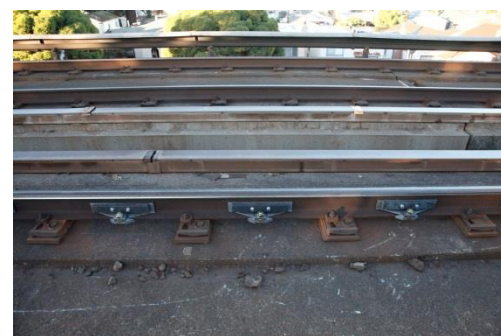
Tuned Dampers on non-ballasted track
